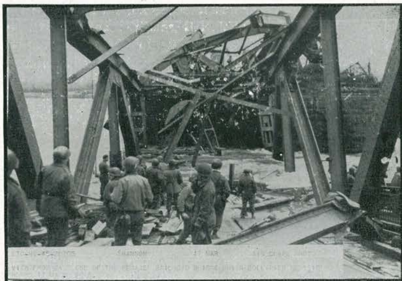
REMGAN BRIDGE SHORTLY AFTER COLLAPSE
