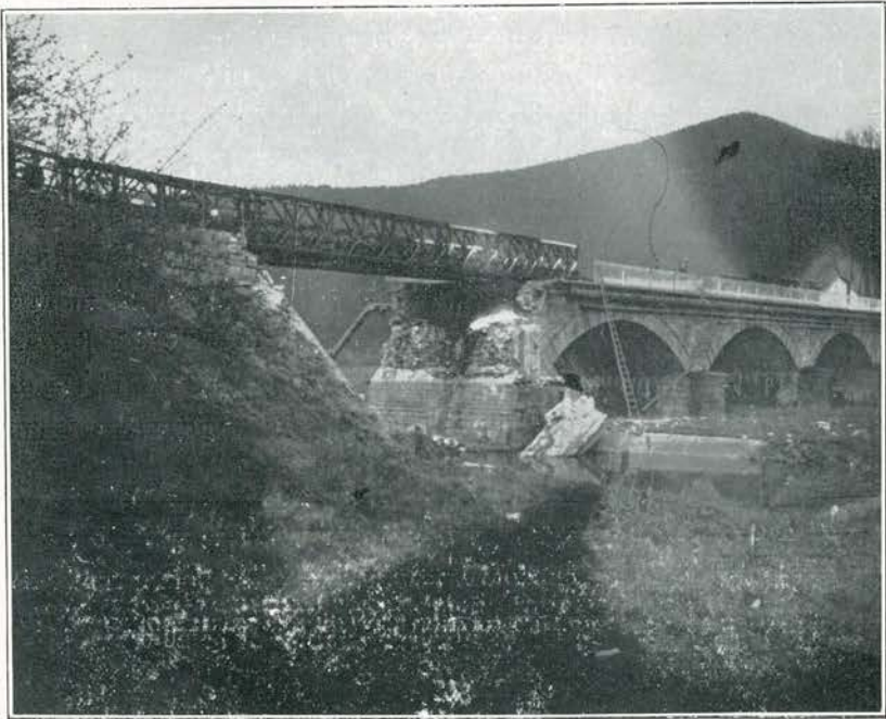
BAILEY BRIDGE AT FREIENOHL, GERMANY
