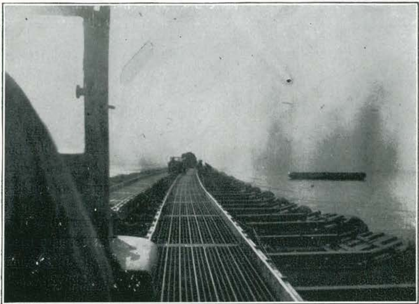
PONTON BRIDGE NEAR HONNEF
