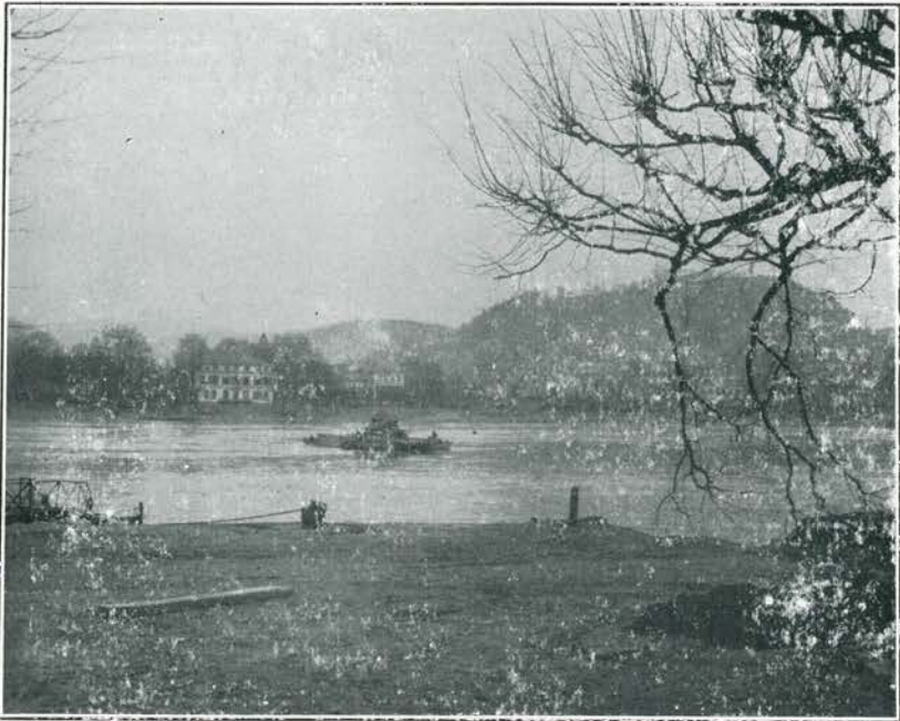
299TH ENGINEER COMBAT BATTALION FERRY NEAR REMAGEN
