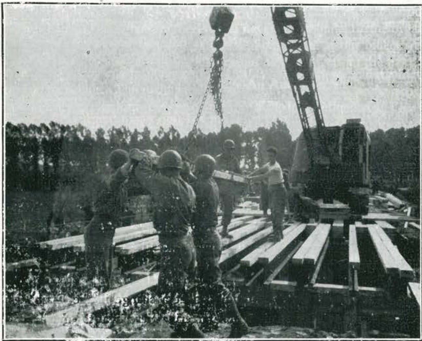
CONSTRUCTION OF STANDARD BRIDGE AT MOXHE, BELGIUM
