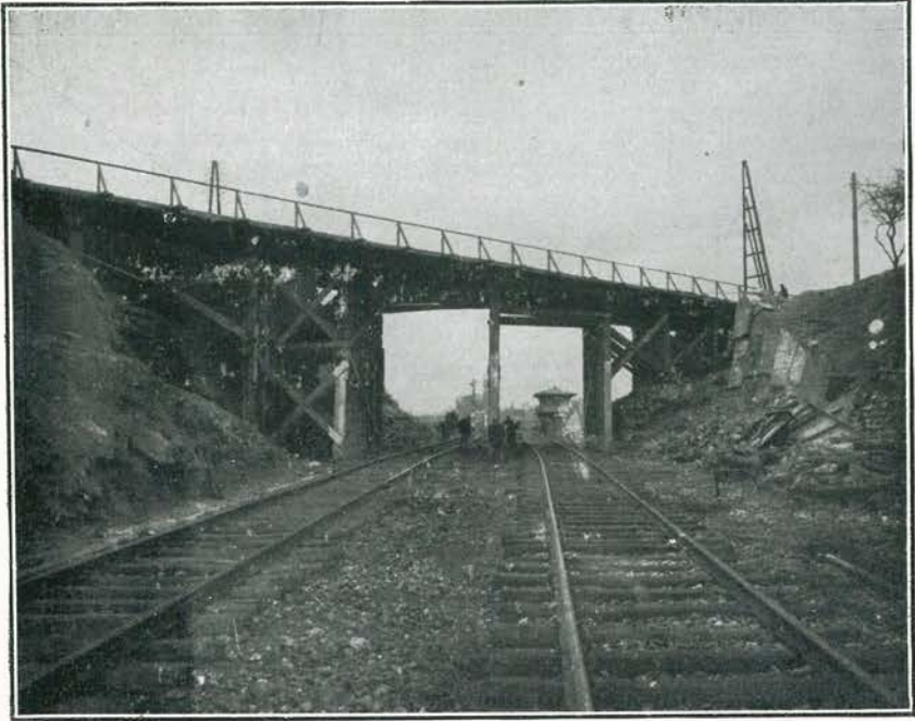
TRESTLE BENT BRIDGE, ARLON
