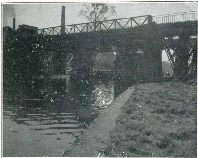
REINFORCED BRIDGES, MAASTRICHT, HOLLAND
